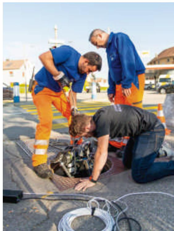
*The workers carefully manoeuvre the high-tech robot into the narrow shaft.*
